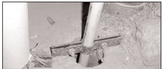
Typical riser supports using FlowGuard Gold® pipe.
