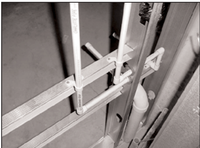
FlowGuard Gold® pipe support at metal studs.
